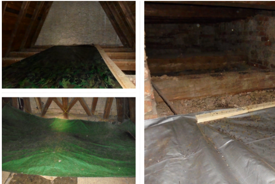
Fig. 3.19: The tarpaulin is anchored with the help of prisms to the collar ties — here, it is sufficient to anchor only at the ends of the tarpaulin — along the tarpaulin is a footbridge made of boards to ensure access during cleaning.
