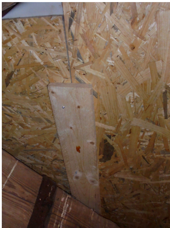
Fig. 3.7: Reinforcement strengthens the boards at the joint. It usually consists of a board placed under the platform at the point where the boards are joined.
