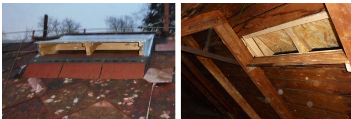
Fig. 6.35: A dormer as a replacement for a missing flight entrance.
