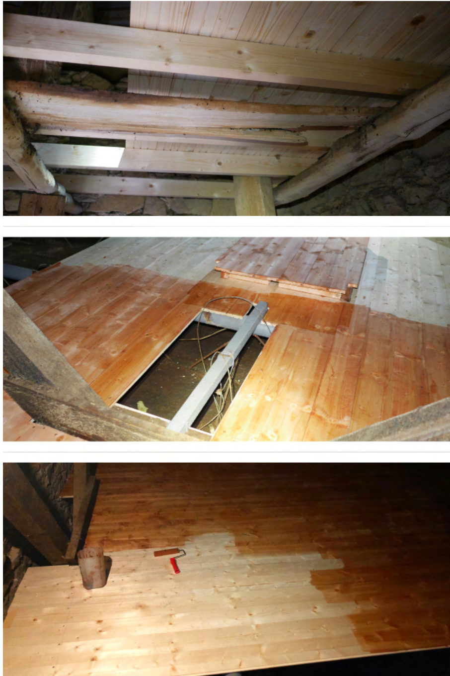
Fig. 3.8: This platform was built in the church tower, where the truss and bells were heavily polluted by guano. Vertically placed prisms were used as a base on which solid spruce boards with tongue-and-groove were laid (↑). The removable part of the platform allows easy access to places where regular inspection or service work is required (centre). We do not need to cover floors made of solid boards with linoleum and foils — they can be treated with a protective surface coating that is harmless to health (↓).
