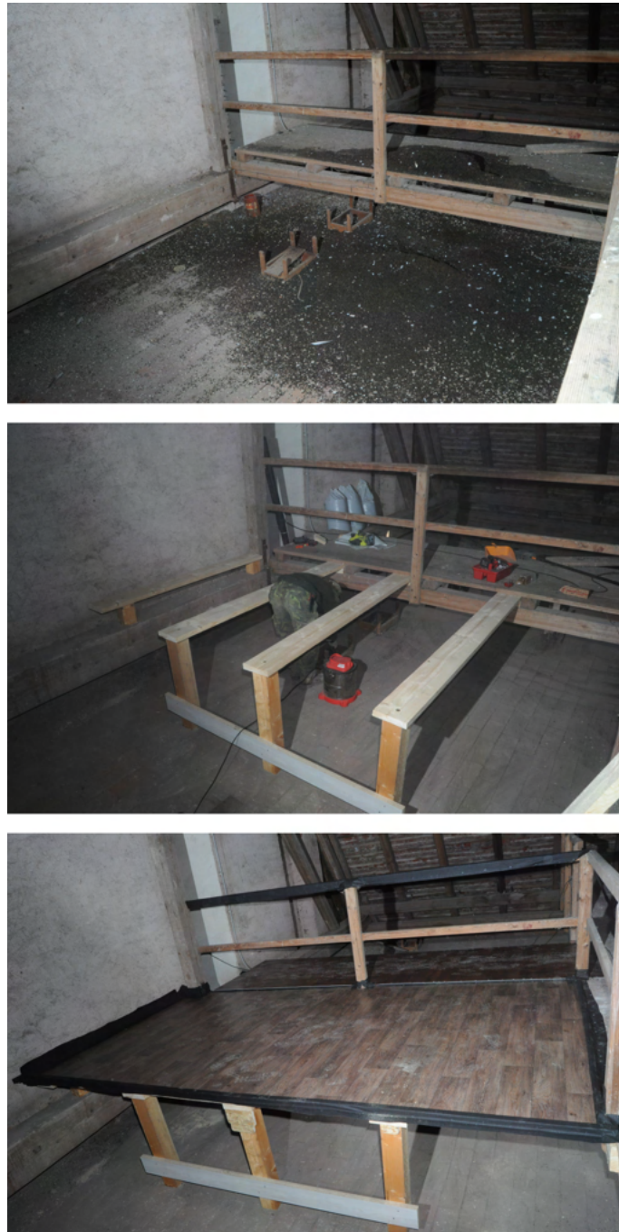
Fig. 6.7: Original state. Guano is on the floor, the catwalk, and the vents (↑). The support structure for the platform is connected to the footbridge. On one side, it is built on uprights (centre). A strip of DTB foil protects the railing. There is a slight height difference between the platform and the technical bridge, which is covered by a strip of DTB foil. (↓).
