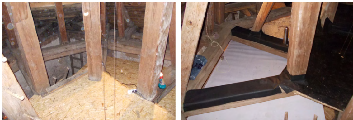
Fig. 6.13: A view of the installed OSB panels in the second and third levels. The same place, but already covered with linoleum (←). The third level is covered with black, and the second with white linoleum (→).
