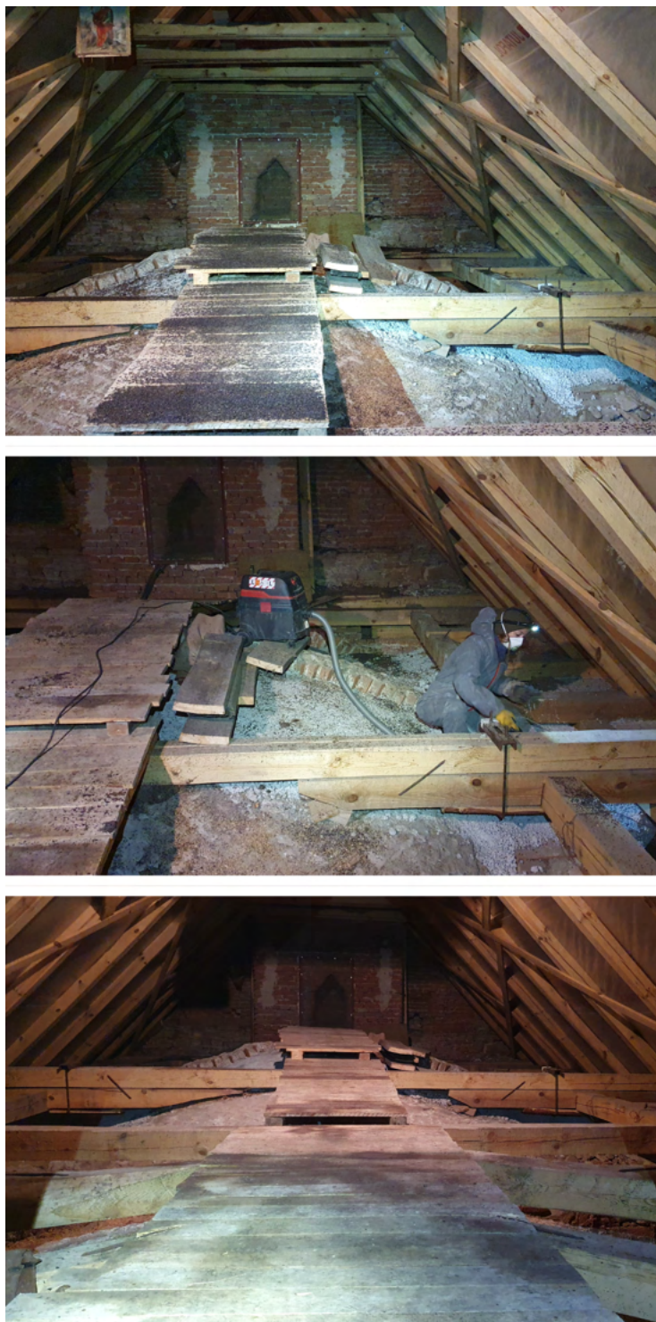
Fig. 6.19: The footbridge and its surroundings are polluted by guano (↑). An industrial vacuum cleaner is a practical tool for cleaning lightly soiled spaces (centre). The resulting state after cleaning the attic and vacuuming the footbridge (↓).
