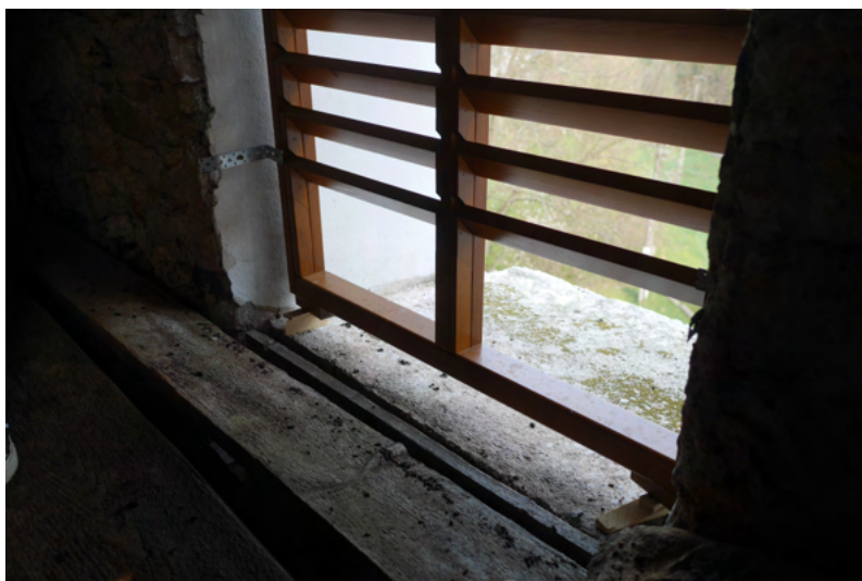
Fig. 6.40: Flight entrance in new window blinds (planned in advance).
