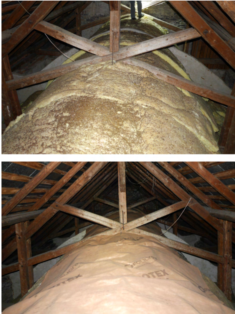
Fig. 6.29: Insulation contaminated by guano. Cleaning such surface is practically impossible (↑). A loosely laid vapour-permeable foil that separates the falling guano from the insulation and facilitates cleaning in the future (↓).
