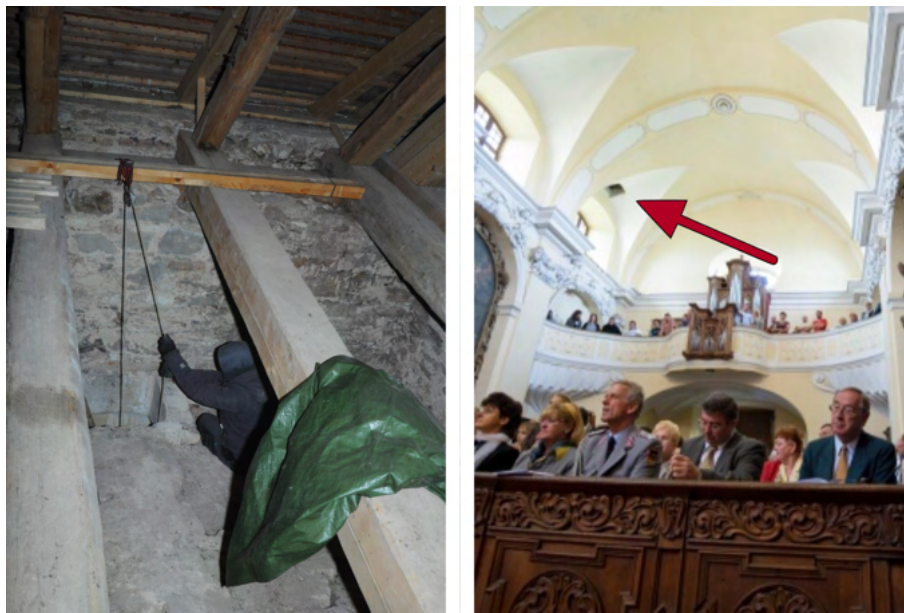
Fig. 6.1: Getting the material to the attic through the small opening in the vault above the choir was difficult. This was done with the help of a pulley and one person on the window sill, who guided the boards so that they passed diagonally through the opening in the vault.
