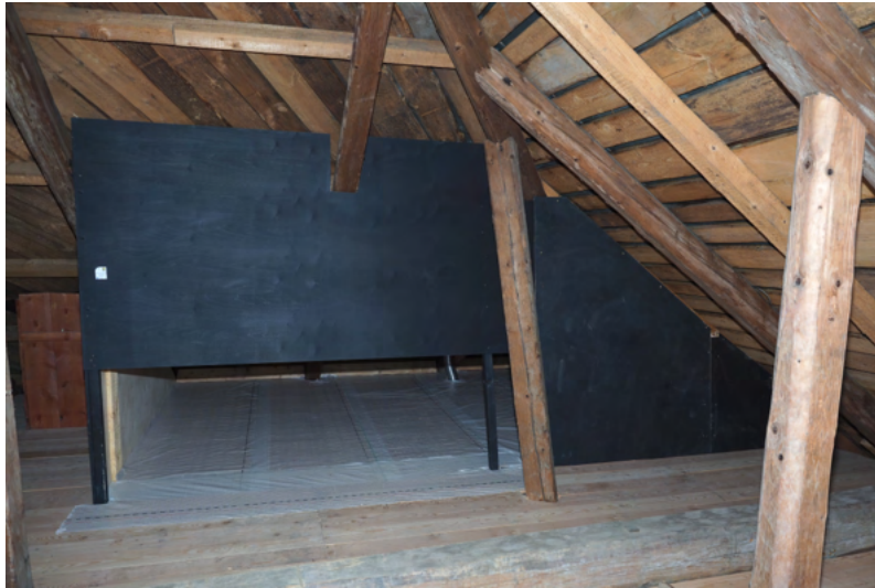
Fig. 6.52: One type of micro shelter in the attic of the abbey is in the form of a small built-in space in a large attic. The floor is protected from guano by vapour-permeable foil (Szczyrzyc; PL).
