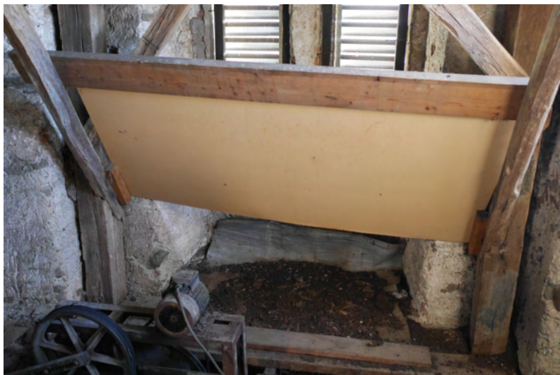
Fig. 6.48: For smaller colonies or in small tower spaces, it is sufficient to divert the impact of droppings. In this case, bat guano falls from a hole in the vault in the church tower onto the floor where the bell mechanism is located. The board is used to deflect the impact of droppings away from these structures - concentrated droppings in this way can be removed more easily (Vyšná Kamenica; SK).
