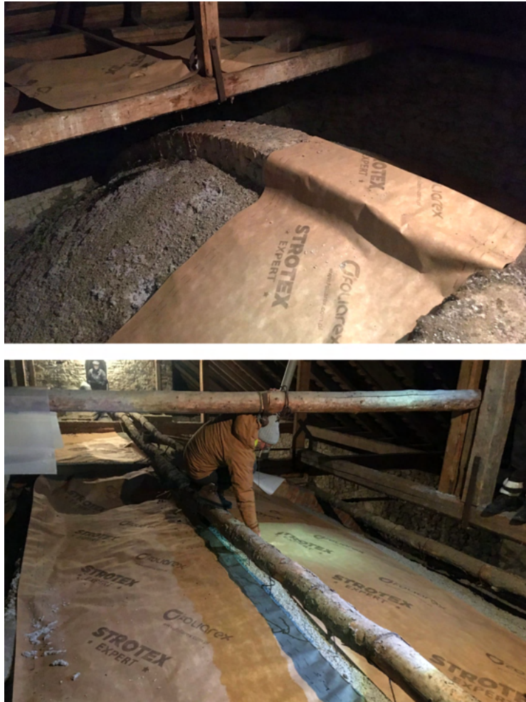
Fig. 6.31: Covering blown-in insulation with a vapour-permeable foil - separates the falling guano and enables cleaning.
