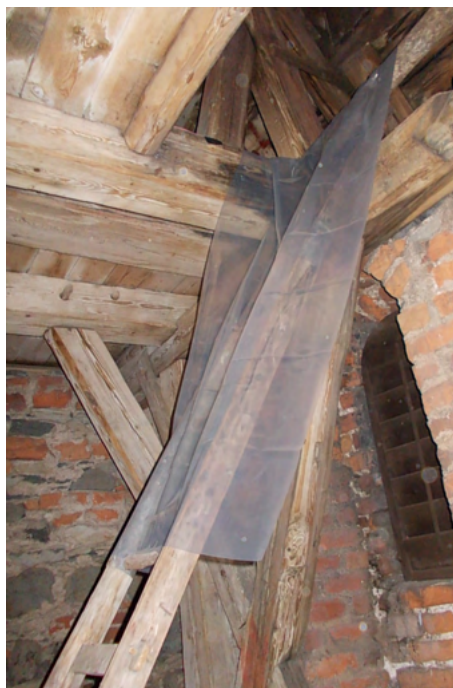
Fig. 6.46: This plastic strip is not installed to trap guano — it has a different purpose. The site had a problem with martens that kill bats. However, the martens could only get to the bats using a ladder. The slippery 1.5-meter-long plastic is an insurmountable obstacle for any marten (Frýdlant; CZ).
