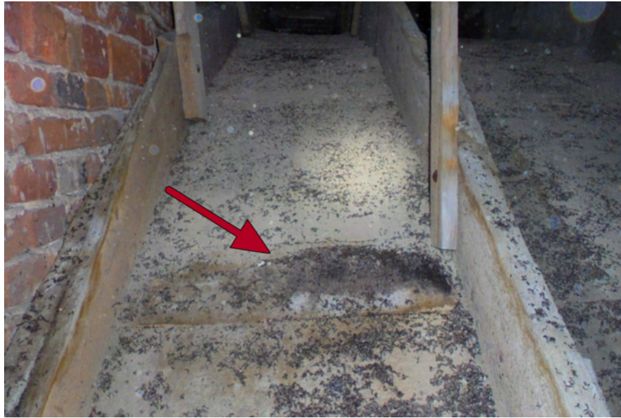
Fig. 1.1: A non-drying layer of droppings on the wooden vault of the church. The church's wooden vault is located under the attic floor. In this church, there is a large colony of the lesser horseshoe bat, about 200 females in size. Any measures are challenging in such a space because walking on the wooden vault is impossible. The only thing that can carry a person safely is a brick ledge along the edge of the wall and wooden ribs made of boards.
