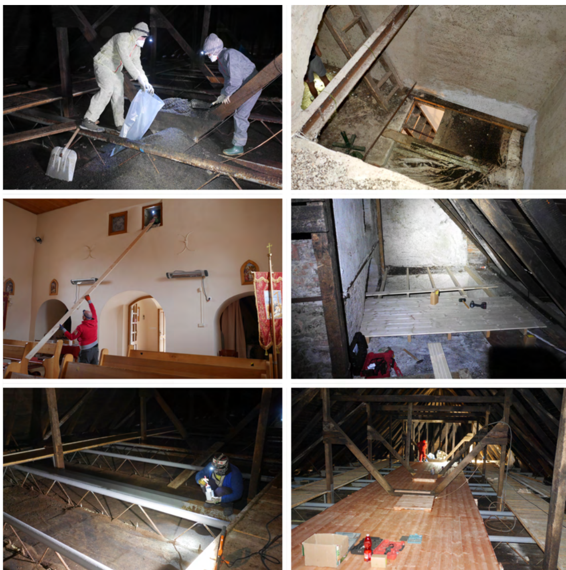
Fig. 6.23: The original condition of the attic. The foil in the background was originally used to catch guano. However, it prevented the necessary air circulation. Also, condensation caused wetting of the insulation. It was removed and replaced with a platform. Construction material were transported into the tower through a small window. The rusting structures were cleaned with wire brushes and treated with anti-corrosion paint. Above the entrance to the tower, a platform made of spruce boards with an area of more than 70 m 2 was installed. It includes two service holes.
