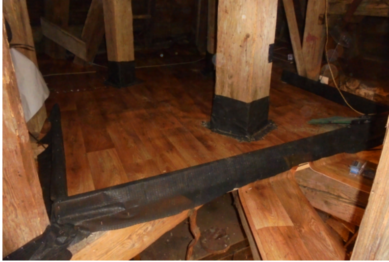
Fig. 6.10: The platform above the clock has a 10 cm wide edge. After the first season, it turned out that the height of the platform edge was correctly estimated. The vertical beams passing through the platform also have a protective collar.
