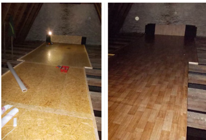
Fig. 6.5: A platform composed of OSB panels laid on beams. The raised edge was created before laying the linoleum (←). Finished platform with soft linoleum bent over a raised edge. The photo also shows the sloping end of the floor near the gable wall (→).
