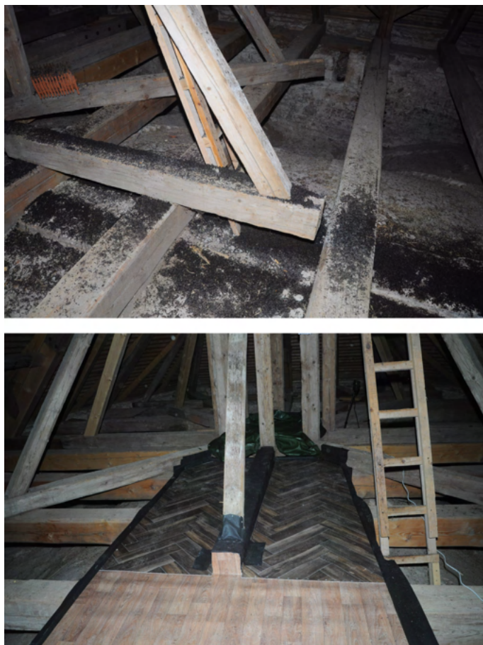
Fig. 6.3: The state before the implementation of measures around the support beam of the tower (↑). The finished platform — the central support beam and the raised edge of the platform are wrapped in DTB foil — the surface is protected by linoleum (↓).
