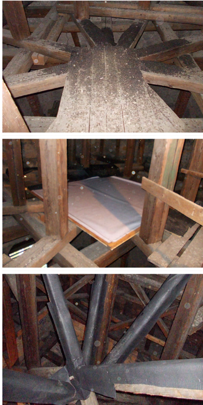
Fig. 6.8: Original state (↑). A simple platform covered with white linoleum catches most of the droppings (centre). Above the platform is a tangle of beams, which had to be protected by strips of DTB foil against guano (↓).
