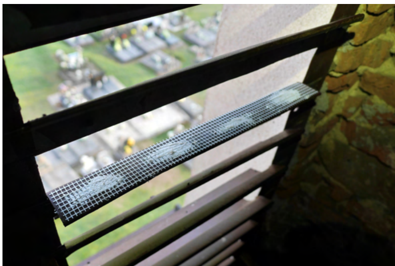
Fig. 6.41: The fibreglass mesh allows bats to land on the blinds. It is glued with UV-resistant glue.
