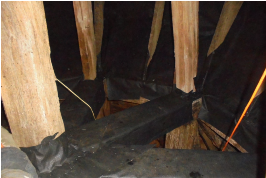
Fig. 3.18: This is an example of using DTB foil to protect places in the tower where bat droppings fall. In addition to the horizontal beams of St. Andrew's cross, the lower part of the tower dome is also covered with this foil.
