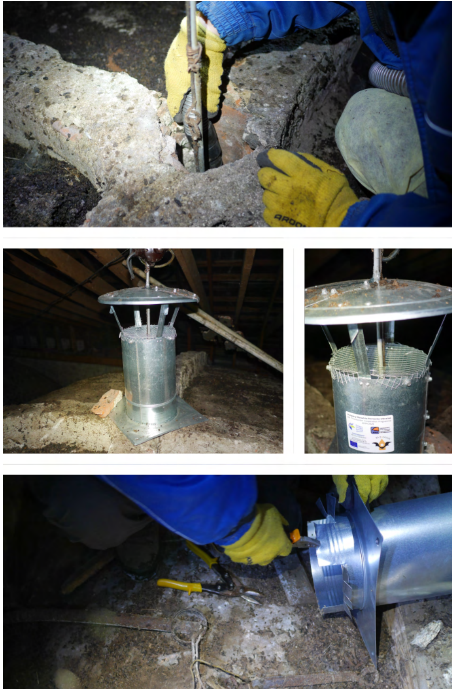
Fig. 4.1: Before installing the canopy, thoroughly clean the opening with an industrial vacuum cleaner (↑). An example of covering an opening with a chimney cap. The pipe must have a thick covering mesh that protects the opening from the entry of bats (centre). We adjust the roof or cover plate on-site using a nailer's tool according to the local circumstances (↓).
