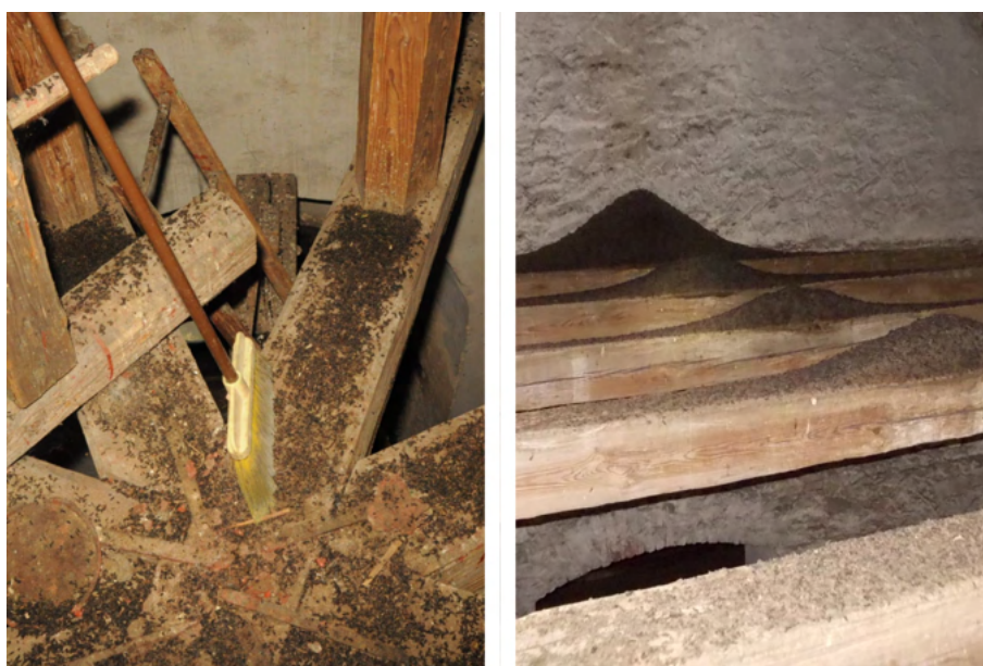
Fig. 2.2: Bat guano dries well in thinner layers, but thicker layers retain moisture. If such a pile is on a wooden structure, it represents a significant problem. In some cases, regular sweeping by broom is sufficient (←). In others, it is necessary to cover the beams with protection (→) after removing the guano.
