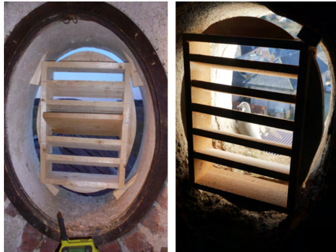
Fig. 6.36: Insert blinds from unplanned boards. The same solution, which effectively prevented pigeons from flying in, was implemented in the attic of the church in the village of Rožňavské Bystré (SK; →).
