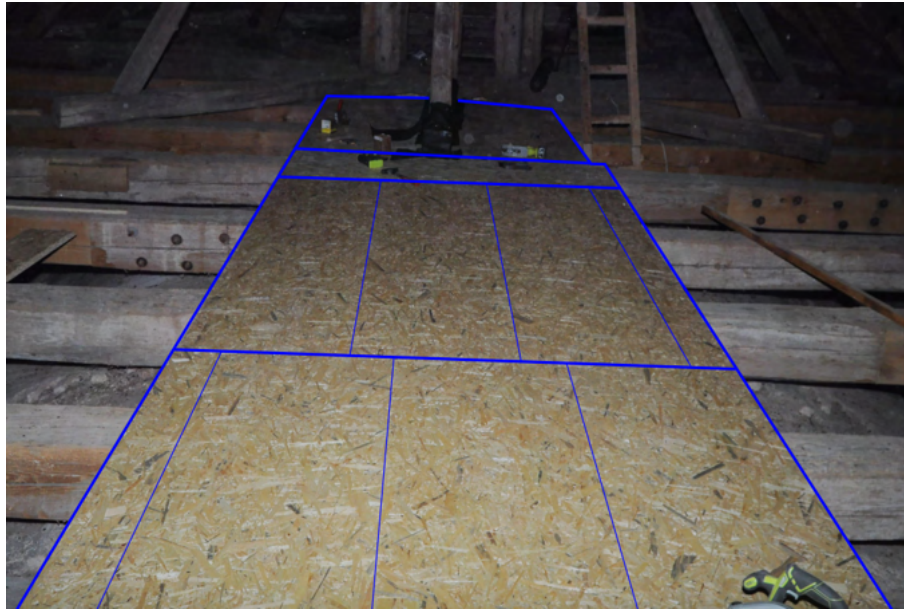
Fig. 3.9: The platform made of OSB panels laid on the horizontal beams in the church's attic. You can notice that three whole panels and one narrow strip are used for the width — it is placed once on the right and then on the left of the platform so that the individual joints of the boards do not connect. The panels' cut can only be on the edge of the platform.
