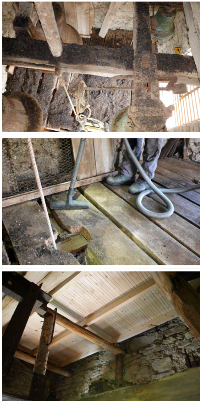
Fig. 6.24: The original state of the church tower contaminated by guano (↑). Cleaning the space under the platform and the bells with an industrial vacuum cleaner (centre). A platform for trapping guano was built above the bell structure (↓).
