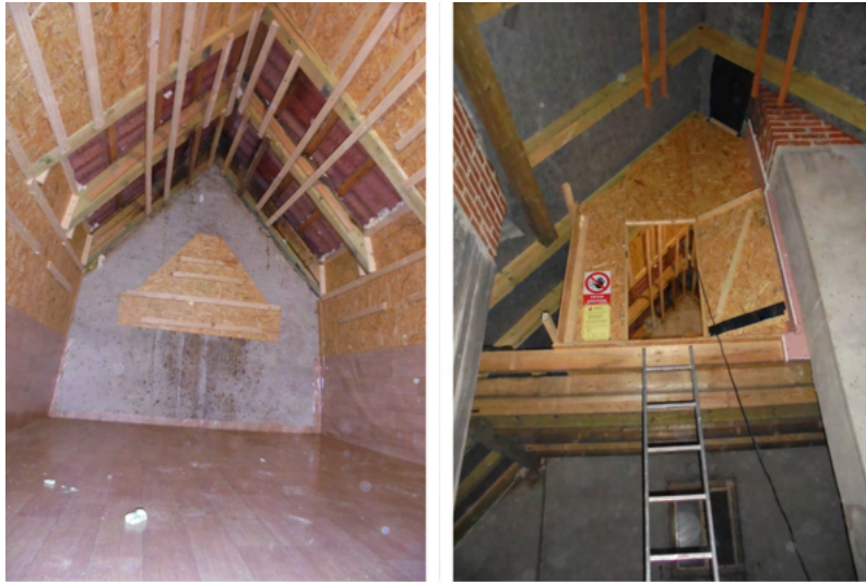
Fig. 6.15: The shed's interior, where the platform is covered with linoleum — in the upper part, there are battens ready for bats to hang. The rear part is warmer and has exposed roof tiles. In the front part, the shed's ceiling is covered with OSB boards so that air flows behind them — this, together with the chimney wall, cools this part (←). A view of the location of the shed on the stilts in the attic. The inventory opening closes and is secured with a padlock (→).
