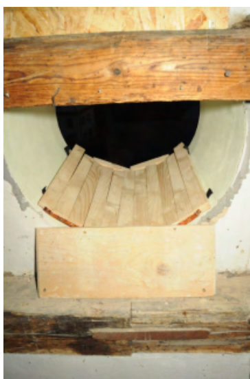
Fig. 6.32: Wooden slatted grate in the circular window.
