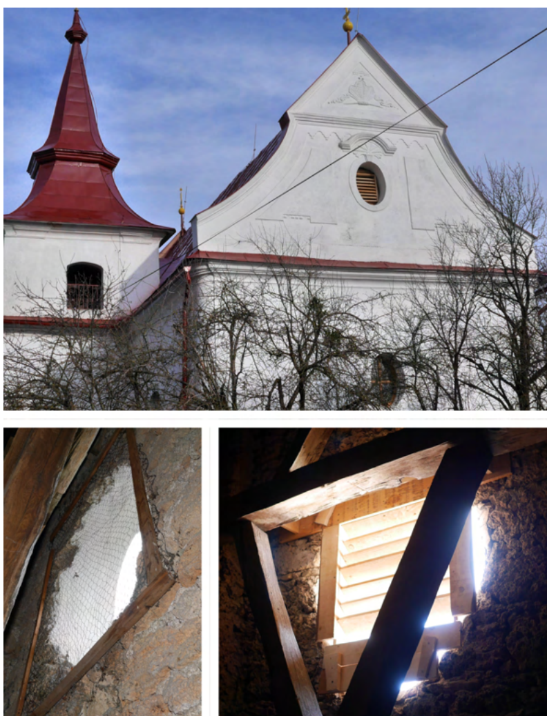
Fig. 6.38: Church in Silická Jablonica (↑). The mesh acted as a trap for bats and caused their deaths (←). Wide blinds made of unplanned wooden boards (→).
