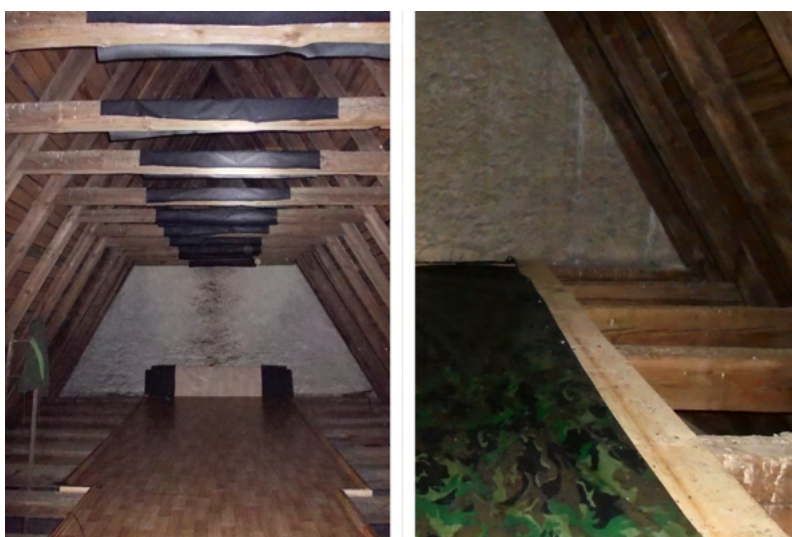
Fig. 6.6: Strips of protective foil on the collar ties (←). A stretched tarp (2×8 m) along which there is a boardwalk to clear the guano.
