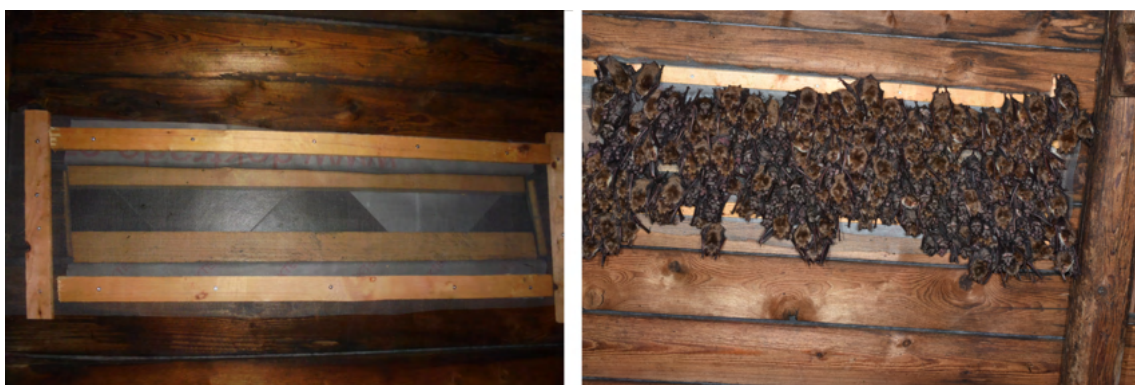
Fig. 6.18: Completed ventilation, where the mosquito net is secured with battens to the original formwork. Already during installation, you could feel the cold flowing air (←). Bats apparently like this measure (→).
