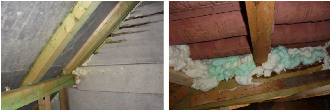
Fig. 6.16: We sealed all the joints with polyurethane foam, even between the gable and the tiles. In this way, bats cannot get into the attic space under any circumstances.
