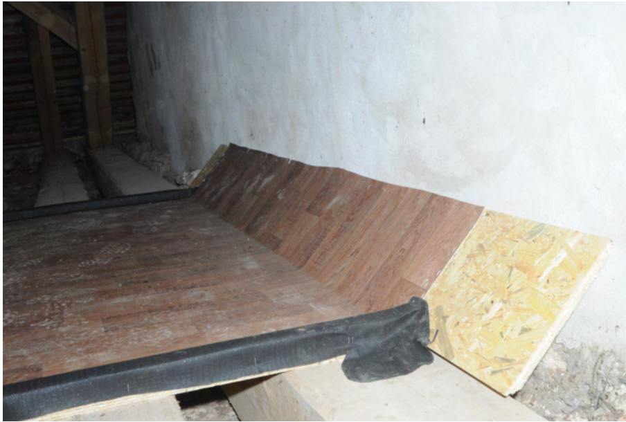
Fig. 3.11: The platform covered with linoleum, whereas it's beginning near the wall is slanted. With such a bend, the linoleum must be carefully pressed into the corner before you attach it, so it does not tear later. A raised edge is already installed on the platform - however, we recommend to install edge later - on the top of the linoleum.
