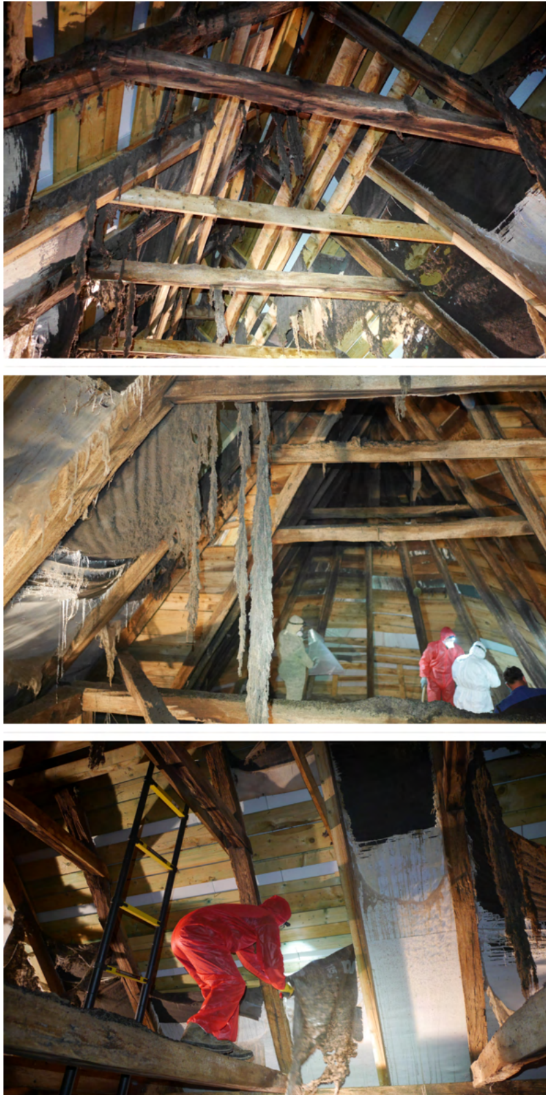
Fig. 6.49: Large bat colonies negatively affect attics, where the vapour-permeable foil is stretched under the roofing. At the same time, they pose a significant risk for bats - they tear them unintentionally with their claws and get caught in the damaged foil. Especially the young ones, they often get entirely entangled and die. This is an example of severe damage to foils in the attic of a church by a colony of the greater mouse-eared bat, the size of 2500 females. Damaged foils had to be removed (Sačurov; SK).
