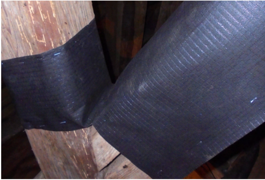
Fig. 3.17: Even in this way, it is very easy to protect the groove of the beam using DTB foil.
