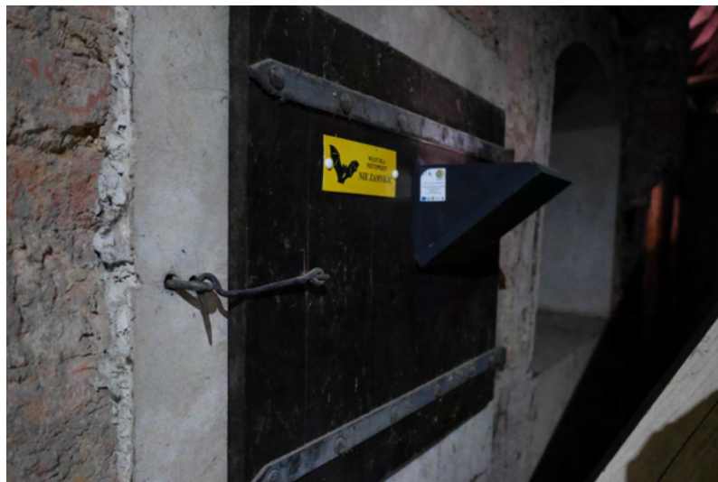
Fig. 6.44: Shade screen on the bat flight entrance. At the same time, the modified flight entrance protects the bat shelter from predators (martens, owls) and prevents pigeons from entering the attic.
