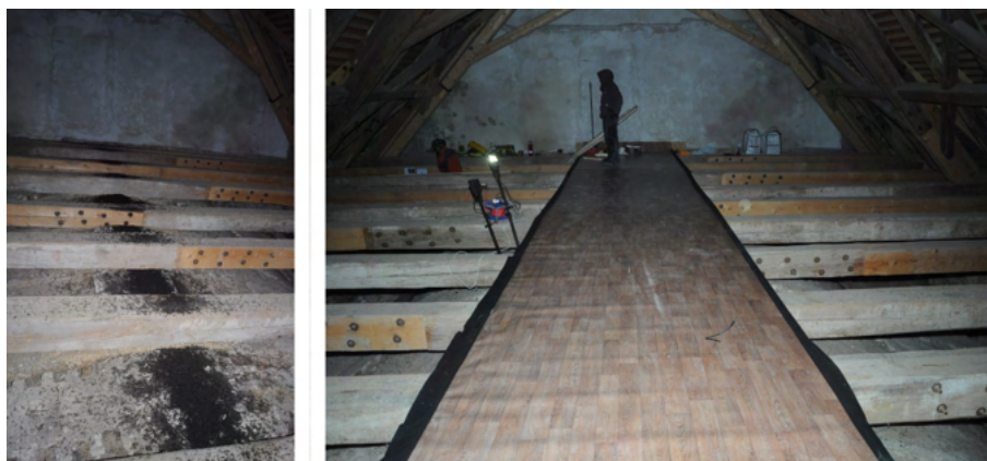
Fig. 6.2: Condition before (←) and after (→) installation of the platform. This measure was implemented very soon after bats occupied the attic. The number of bats and guano is small. The platform's capacity is also sufficient for a larger colony of bats. If the number of bats does not increase dramatically, cleaning is only necessary once every three years.
