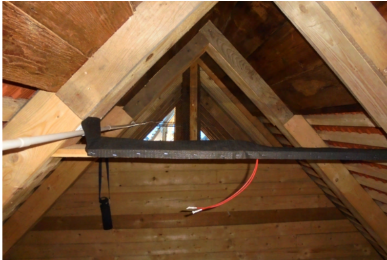
Fig. 6.47: Electrical installation, fire detectors — if installed under bats, they are very difficult to clean. It is, therefore, advisable to cover them with DTB foil (Horná Police; CZ).
