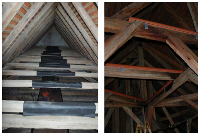
Fig. 3.16: Protection of collar ties above the platform using a strip of DTB foil (←). Alternative solution with split PVC pipes (→).
