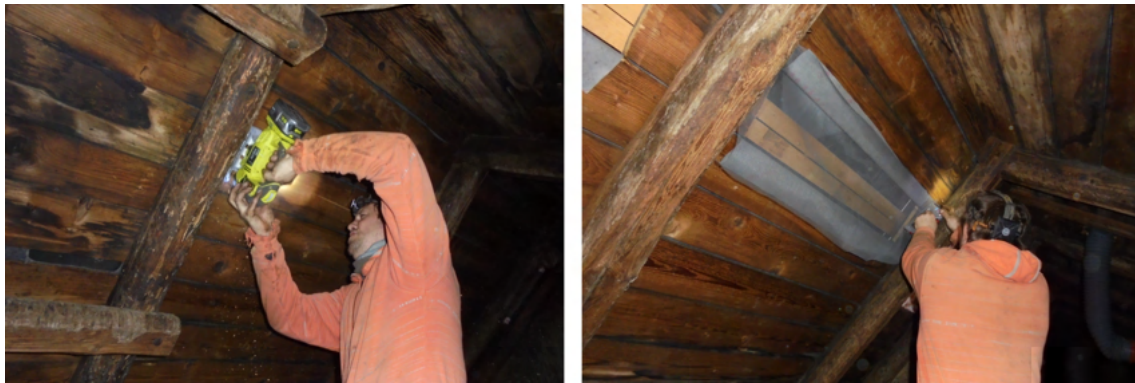
Fig. 6.17: Cutting the original formwork with a jigsaw (←). It was necessary to cut and secure the vapour-permeable foil (→).
