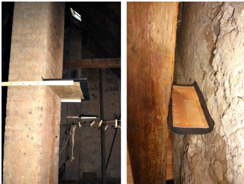
Fig. 6.45: On hot days, bats like to cool off on walls and the walls of chimneys. To reduce the amount of guano on the floor, an OSB panel can be attached to the chimney using laths and dowels (Vysoké Veselí; CZ; ←). If the stand is too close to the wall and it is difficult to clean behind it, we can use an additional board in the place where the gap widens (Horná Police; CZ; →).
