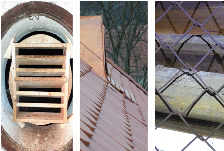
Fig. 4.3: Blinds installed in the flight entrance prevent pigeons from entering. These blinds are fixed only with small wooden wedges — thanks to this, bats can also climb the wall around the blinds (←). A slatted grate located at the flight entrance of a large bat colony on a new glazed roof covering (centre). Rusted mesh does not cause any problems for bats when climbing (→).
