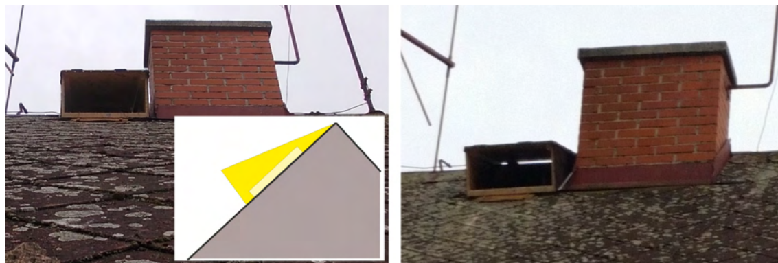
Fig. 6.34: A hinged dormer allows bats access to the attic.
