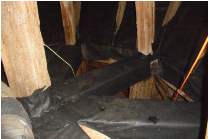
Fig. 6.11: In the highest level of the tower, the beams are covered with DTB foil, and the formwork of the tower's dome in the lower arch is protected in the same way.
