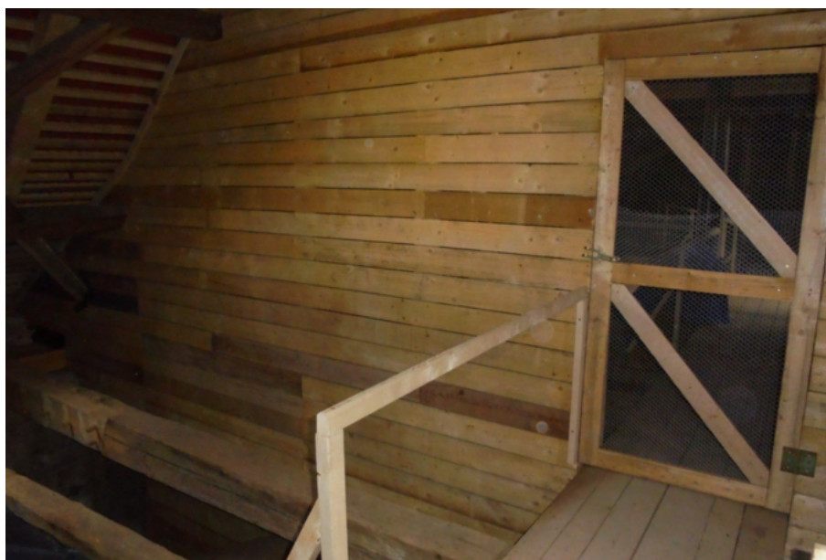
Fig. 4.2: Partition of the attic space with a board wall. A mesh in the door and near the shield ensures natural air flow - the microclimate, therefore, remains unchanged.
