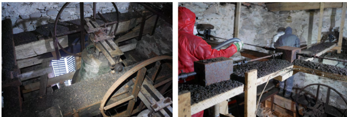
Fig. 6.20: Original condition — guano pollution is severe and damages the wooden structures and the mechanism of the bells.
