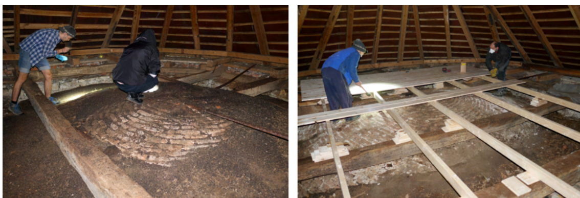
Fig. 6.26: The original contamination of the vault and its surroundings by guano (←). Foundation of the platform and adjusting its height above the vault (→).
