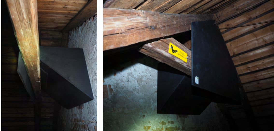
Fig. 6.43: A shelter constructed of wooden boards with a dark coating in the attic of the Cistercian Abbey, including a shading screen for the shelter's interior.
