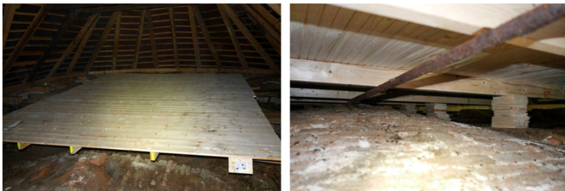
Fig. 6.27: The finally assembled platform in the back part of the attic - the place where the colony of bats gathers (←). Underpinning the prisms with columns from board scraps (→).
