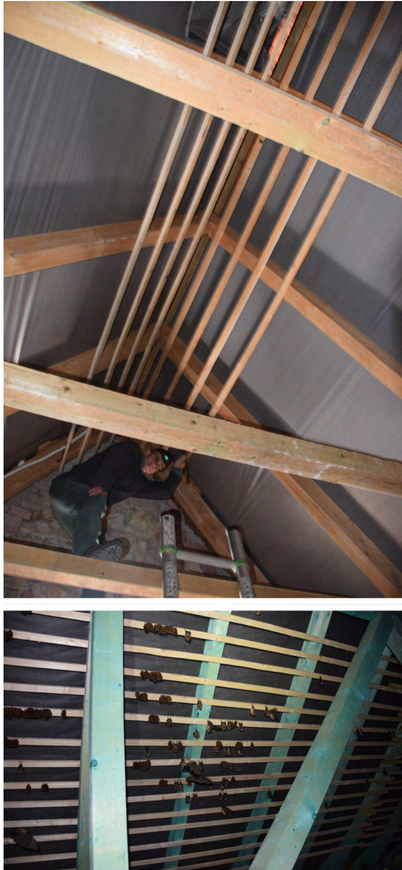
Fig. 6.50: The habitat choice of bats in the attic can also be guided by the additional construction of elements for holding and hanging individuals. In this case, it involved the installation of battens from the underside of the rafters so that bats do not damage the vapour-permeable foils. This measure can be efficient and effective, for example, in colonies of lesser horseshoe bats.
