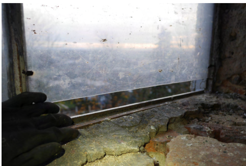
Fig. 6.42: Flight entrance reduced by plexiglass.
