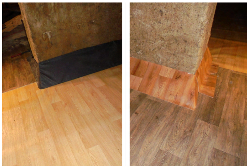
Fig. 3.14: Diagonally laid boards protect chimney - they are around the entire chimney (←). The boards are covered with DTB foil, on which a strip of linoleum is still attached (→).
