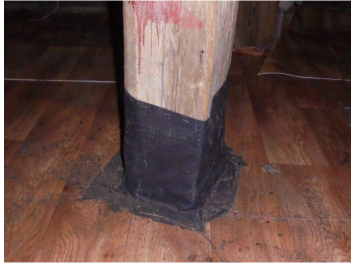
Fig. 3.15: Protective collar made of DTB foil on the vertical beam passing through the platform.
