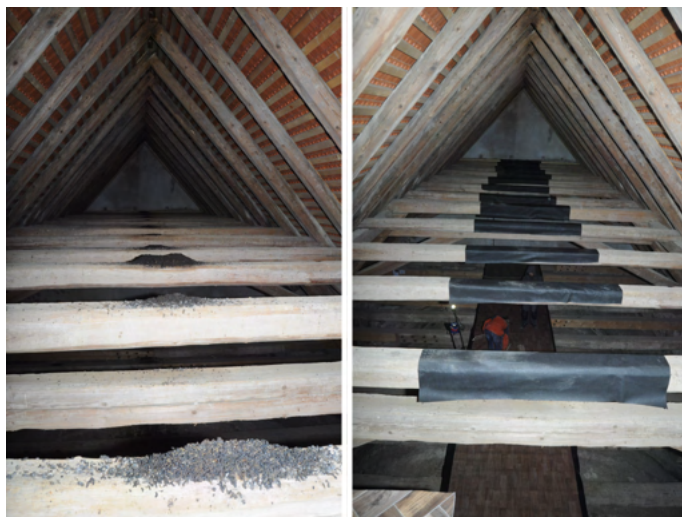
Fig. 6.4: Bats often hang on the rafters under the ridge, so a large amount of droppings is caught on the collar ties (←). Simple protection of the collar ties using a strip of DTB foil attached to the beams with a stapler (→).
